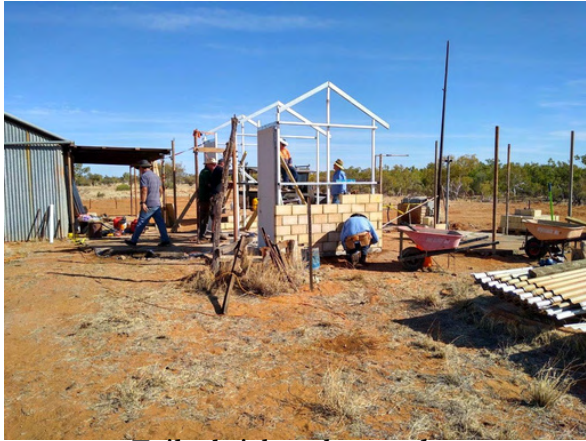
Toilet brickwork started
