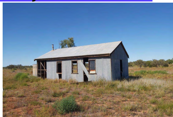
Old Shearer's Shed & Dining Room before restoration
