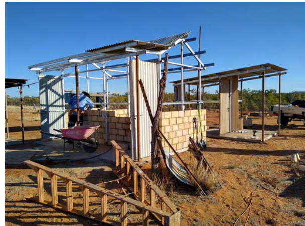
Toilet doors on & shower frame up
