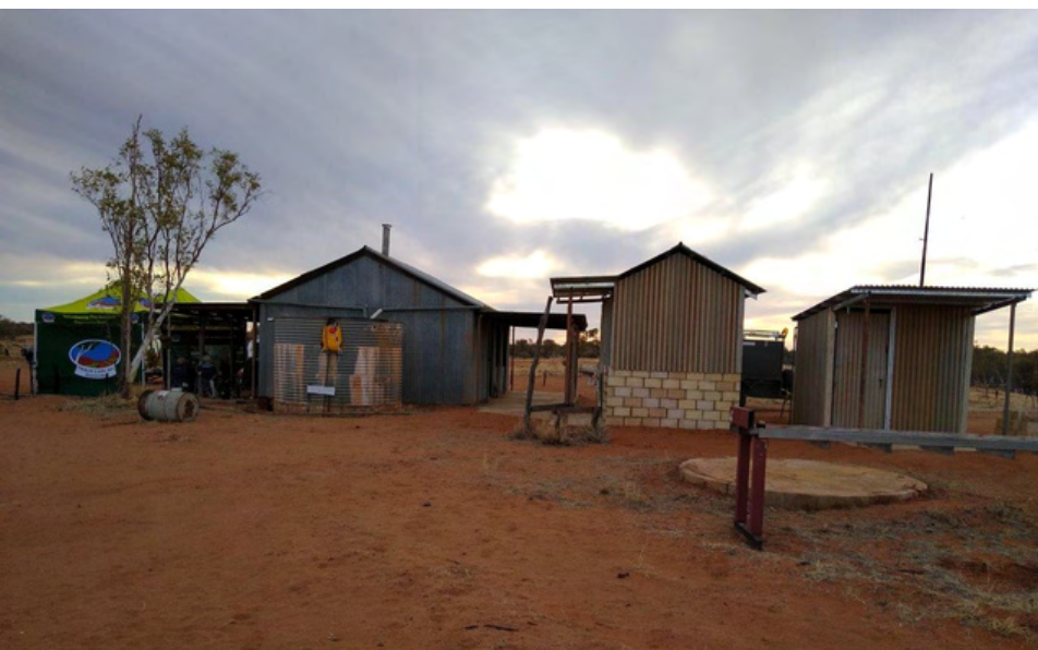
Completed toilets & shower
