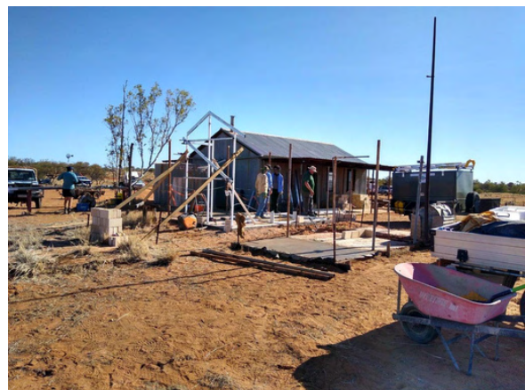
Toilet Framework started
